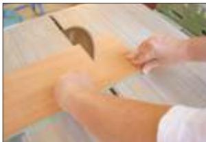
Step-by-step: The end of the stair rise will be cut in a 45° angle.
