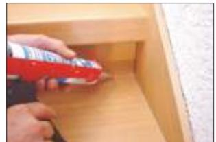
After the step and the stair riser are fixed you have to close the rabbet with coloured silicon.
