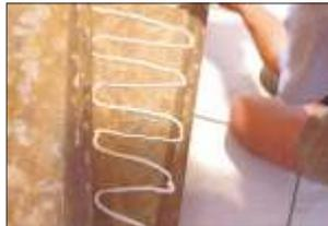
To fix the step you just put the special glue in snake line on the old and the new step.
