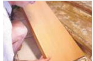
The new step has to be put down and pushed back with the fist or a special hammer.
