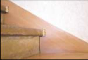
The string board will be cut out of a board, like a panel or polyester board, and just glued on.
